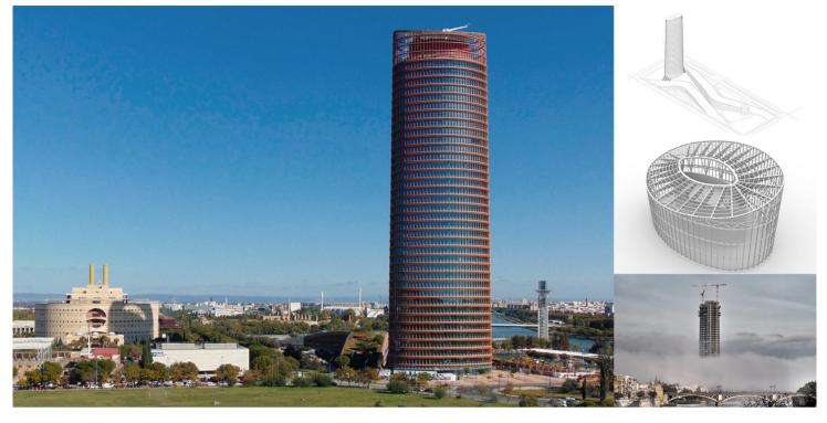
The Seville Tower, designed by the architect César Pelli, is set within the boundaries of the Triana Port complex in Seville. The building is 180.5m high composed of 38 storeys above ground level and 3 below. The plan elevation is elliptical, measuring 52.0m by 36.0m.
